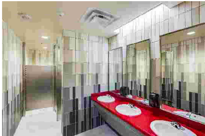
Newly renovated restrooms
